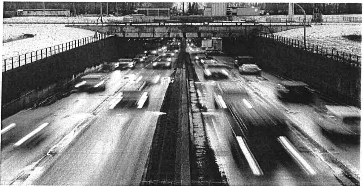
Early-warning technology for earthquakes, developed by a Vancouver-based company, uses sensors to detect the first seismic waves, analyze them and, if necessary, shut down traffic into the George Massey Tunnel. RICHARD LAM/FILES
