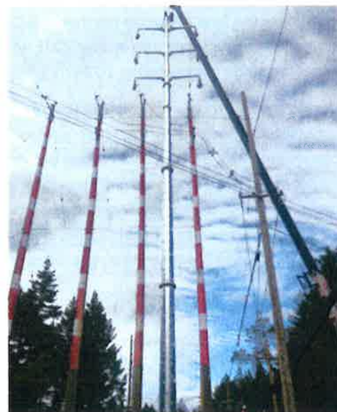
Mudge Island 2019 – old and new. The newly raised steel monopole in close proximity to the four pole wooden structures.
