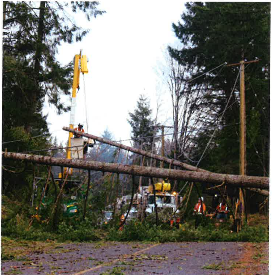
Crews undertaking restoration and repair work in Nanaimo.
