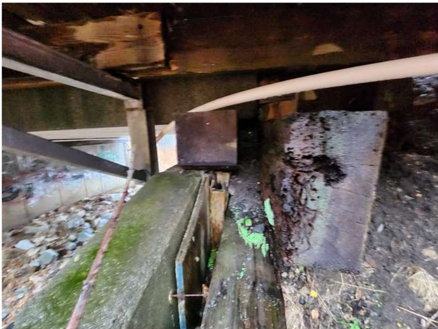
14 - Typ. Upstream Ballast Wall at Pedestrian Walkway
