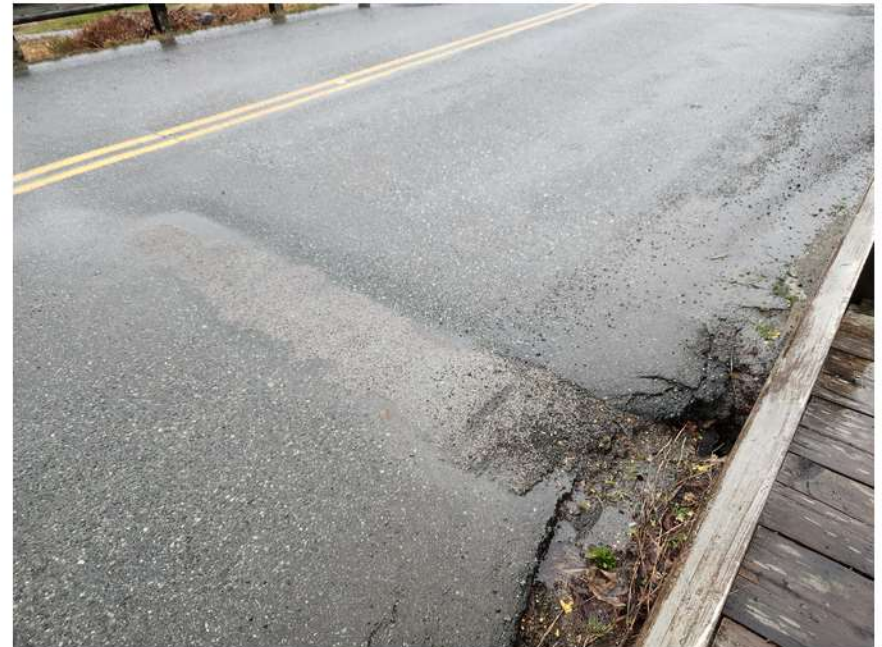
08 - Fill Settling Sound Abutment
