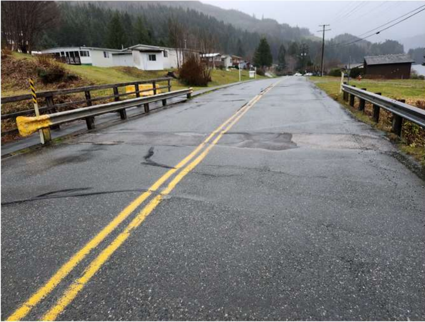
09 - Fill Settling North Abutment
