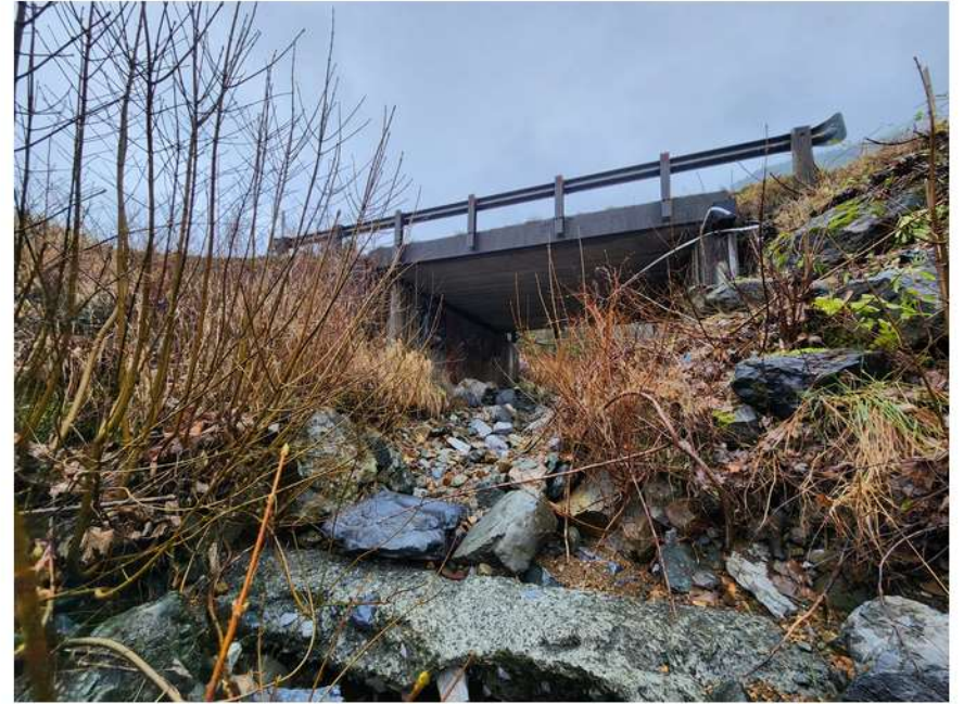
10 - Downstream Riprap Weir
