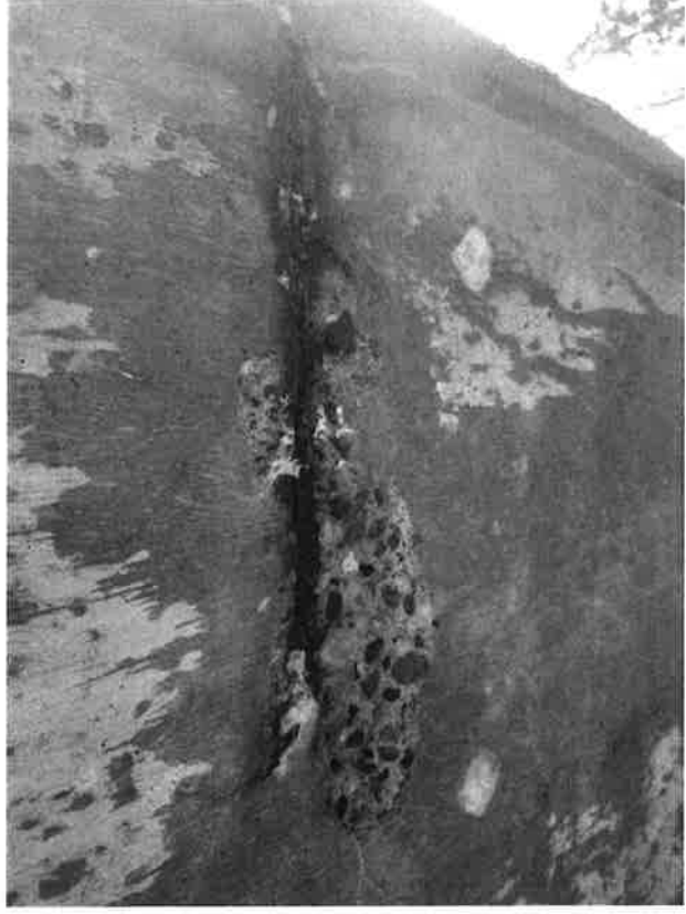
10 - Rebar Corrosion
