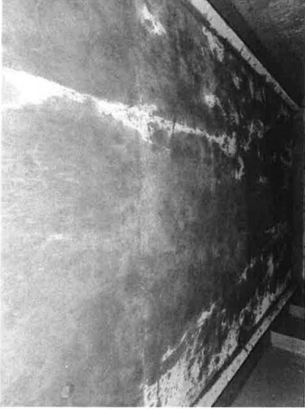
16 - Typical Underside of Deck
