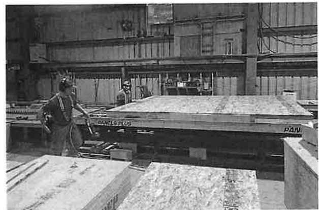
RAS employees assemble a panel at their Chemainus facility, which will then be sent to the build site at NIC’s Comox Valley campus.
