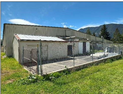
Photograph 5: Rust to roof cladding of shed.
