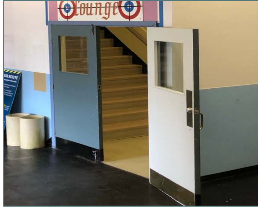
Figure 21: Glazing at interior doors
