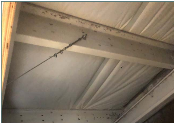
Figure 1: Roof insulation, blanket type
