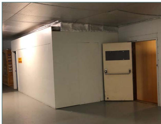
Figure 8: Concourse Change Room
