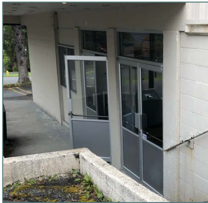
Figure 16: Glazed Entrance Doors
