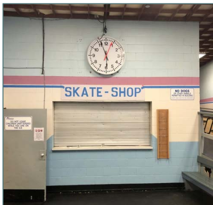
Figure 10: CMU fire wall
