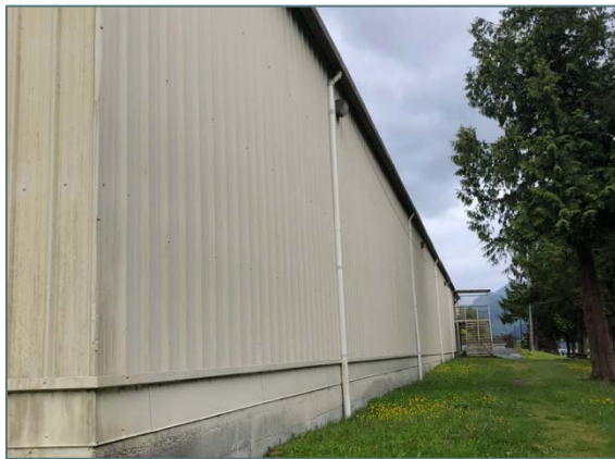
Figure 4: Exterior corrugated metal siding
