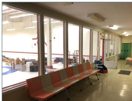
Figure 19: Glazing at Curling Surface
